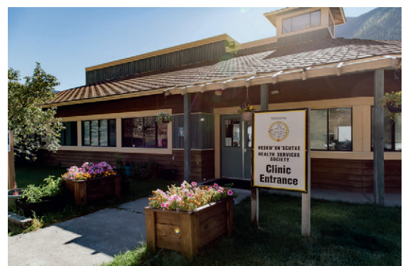
HHSS Office / Clinic at Spences Bridge
